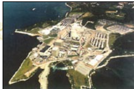
Millstone's site in November 1999
